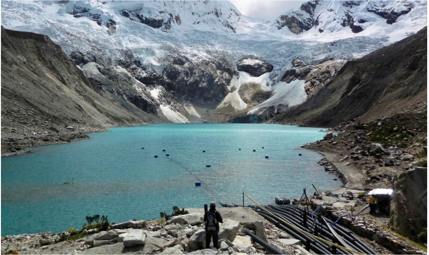
Pictured: Syphoning for lake level lowering and flood protection at Laguna Palcacocha, Cordillera Blanca, Peru. Rock and ice avalanches from the surrounding icy peaks can directly impact the lake. Photo credit: H. Frey, April 2015.
