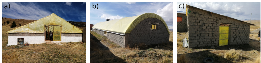
Figure 2. Photographs illustrating the different greenhouse roof types used by local farmers: (a) two slopes, (b) semi spherical, (c) single slope. These images correspond to greenhouses 1, 22, and 25, respectively (see their characteristics in Table 1).
