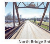
North Bridge Entry
