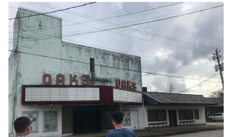
Buildings need to be renovated
