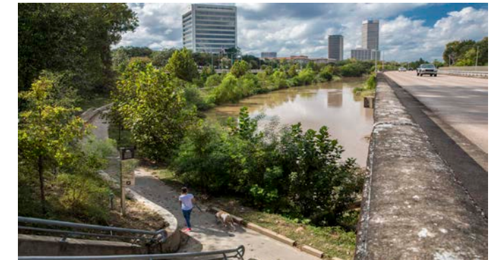
Pedestrian Stairs - Post Flood
