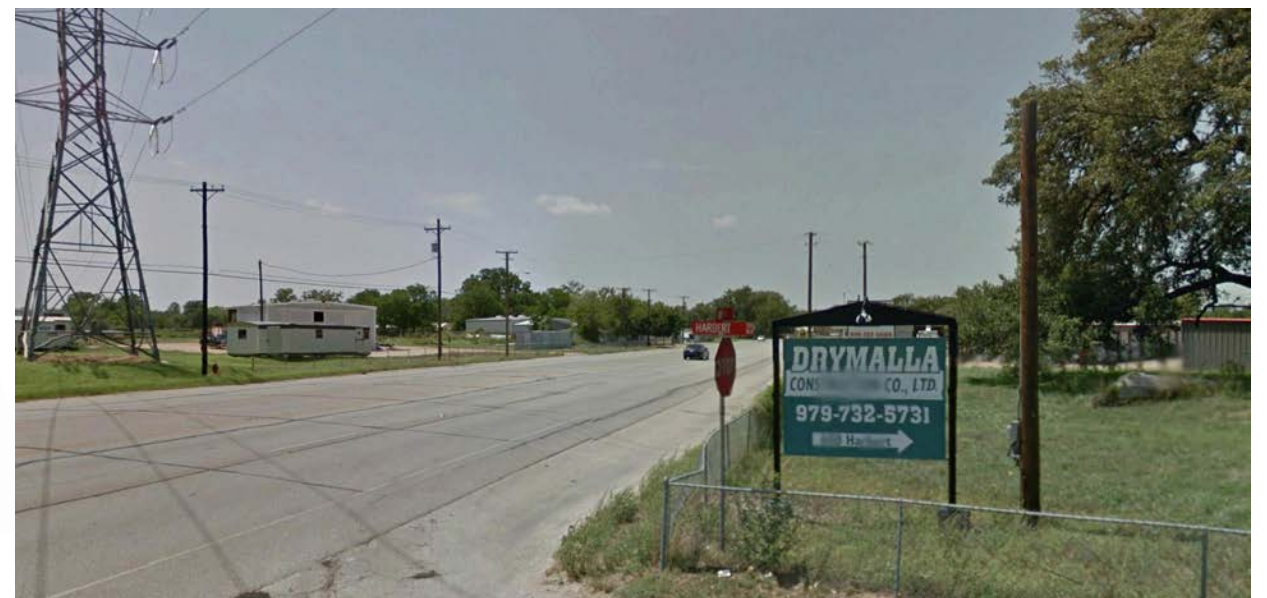
Existing - Houston St. Intersection
