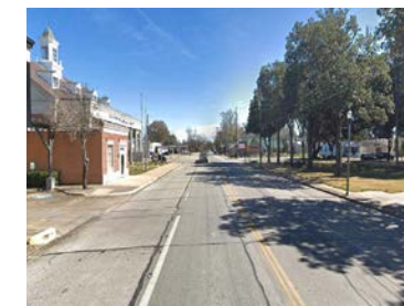
Existing streetscape conditions
