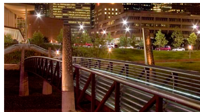
Bridge Lit at Nighttime
