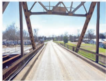
North Bridge Entry
