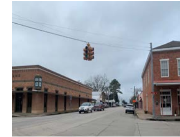
Existing streetscape conditions
