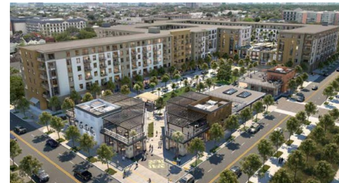
New apartment complex breaking ground at West Dallas and Dunlavy
