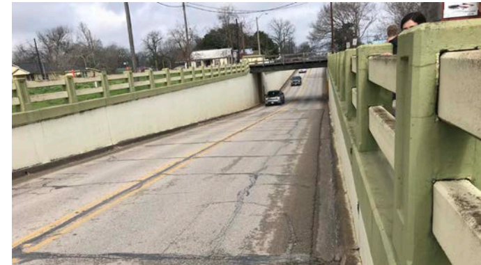
No shoulders or sidewalk
