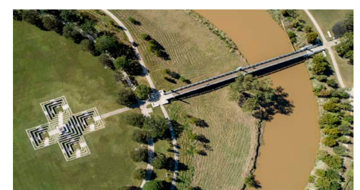
Gabion Edge/Pedestrian Bridge - Post Flood
