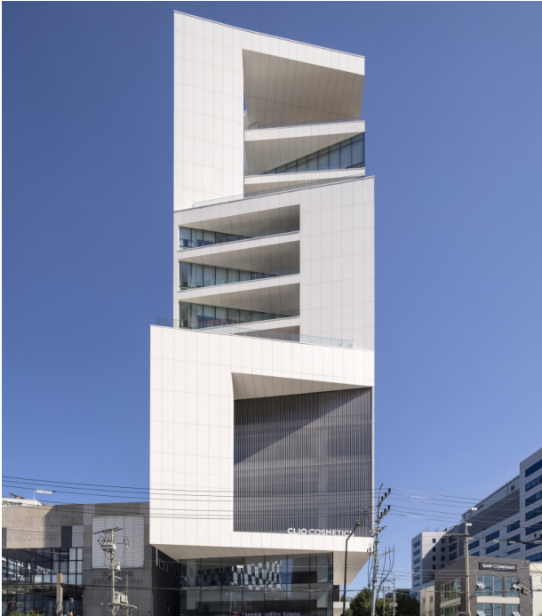
Figure 46. Clio's new office building that uses terraces as a design and experiential element. Image source: Namgung, n.d.
