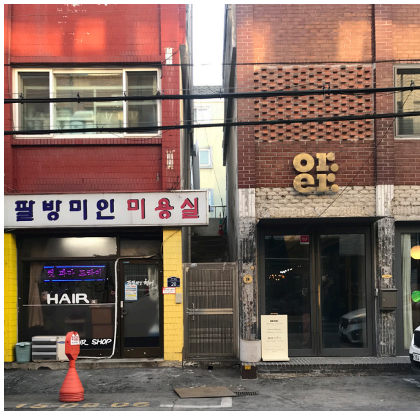
Figure 17. OrEr repurposed a low density mixed-use building (commercial, industrial, and residential) to create a multi-floor cultural space that hosts exhibitions and seminars and a cafe on the first floor. This pictorial layout that shows an old-timer hair salon, still operating, next to the new space is a popular image on social media. ([Seoul Hiptown Tour -Seongsu-dong edition-], 2019) Image source: author, 2020.
