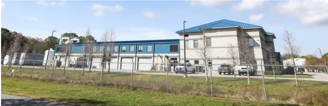
Figure 2-1 Oldsmar's Bruce T. Haddock Water Treatment Plant [11]
