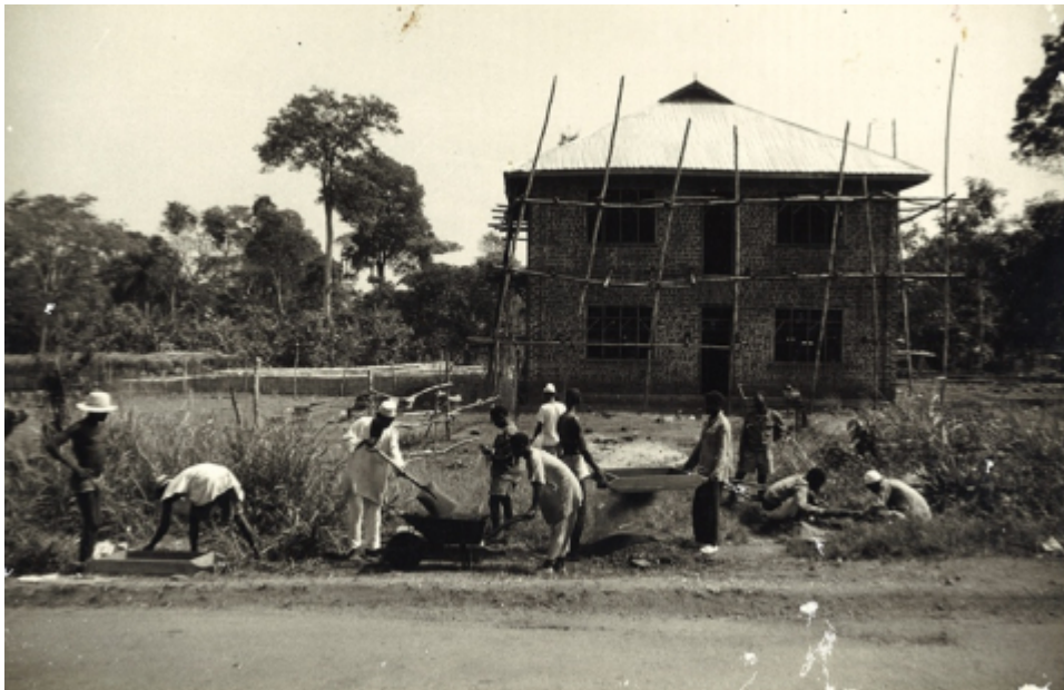
Figure 4 – "Almost-completed one-story house," ca. December 1957.
