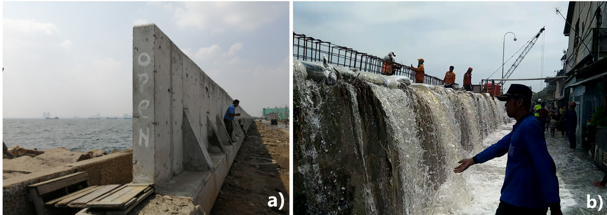
Figure 5. Sea Dyke in Jakarta: (a) the newest sea dyke; (b) the flood overflowed the dam.
