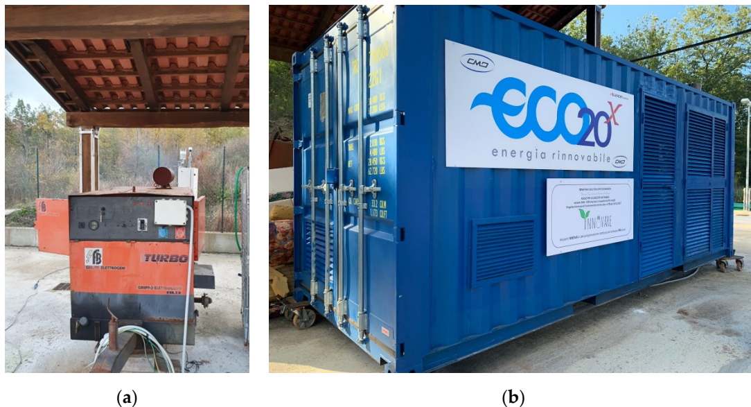
Figure 23. Traditional diesel oil-powered generation set (a) and CMD ECO20X unit (b).
