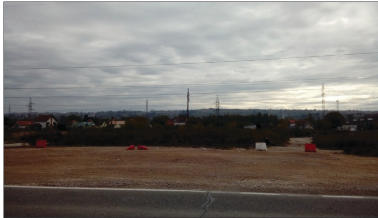
Figure 2 - Evicted residential buildings and space intended for the expansion of the surface mine in the settlement Vreoci
