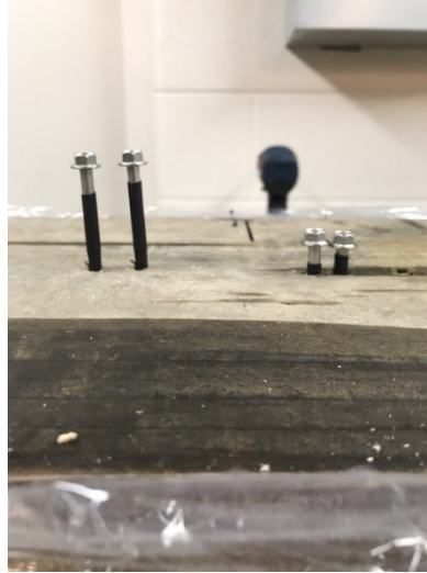
Figure 2.5 Insulated screws used to check moisture content of specific layer in CLT.
