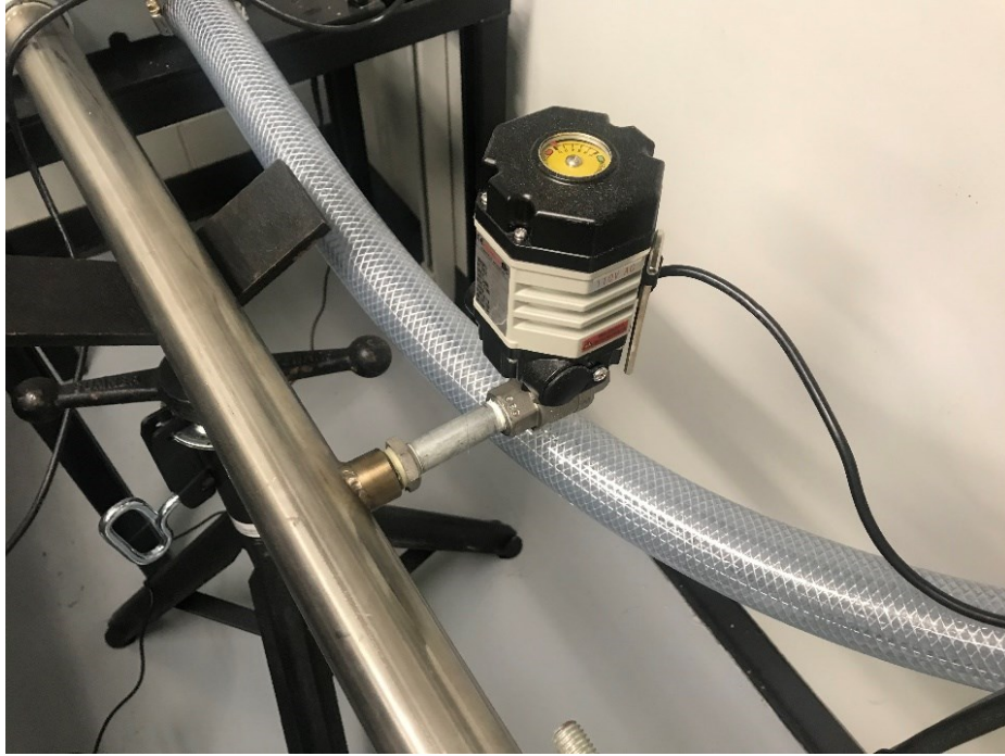
Figure 3.33 Make-up Air Valve and Actuator
