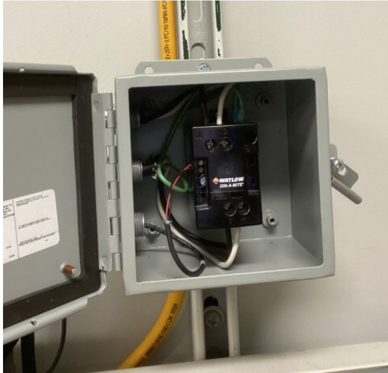
Figure 3.5 Heater Relay Controller.
