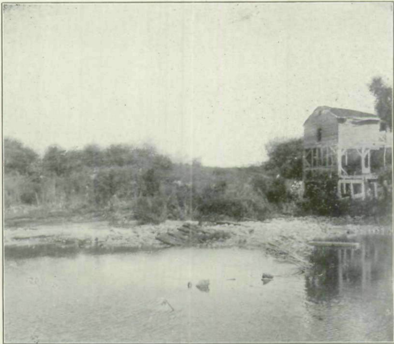
THE HEDDLESTON-SIGLER-COLTRAIN MILL, CEDAR TOWNSHIP.
