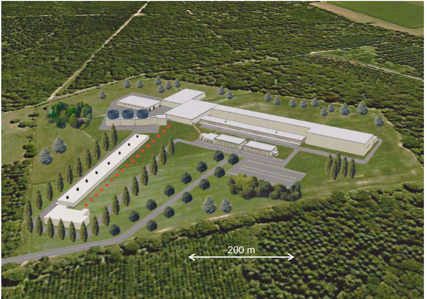
Fig. 2: Proposed layout on a “green-field” site. The driver accelerator (240 m long) is located beneath the red discs.
