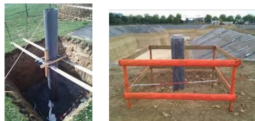
Figure 3: Pillar under construction and protective fencing around geodetic pillar
