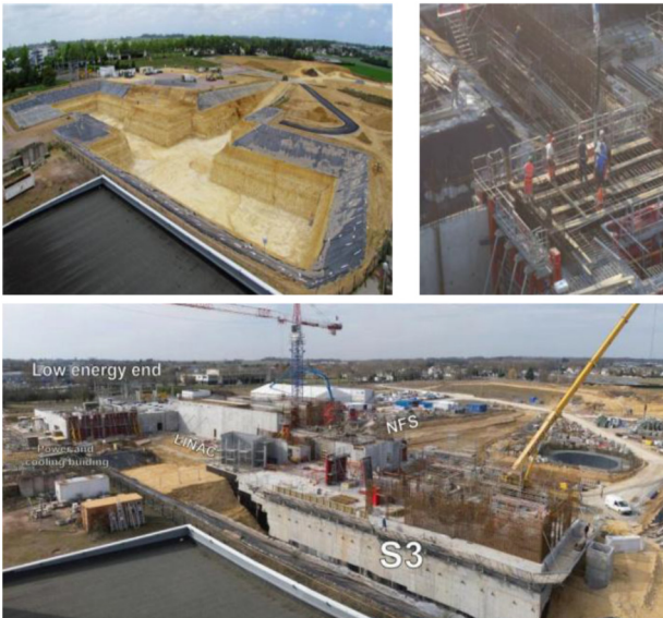
Figure 6: Views of the construction site under way.
