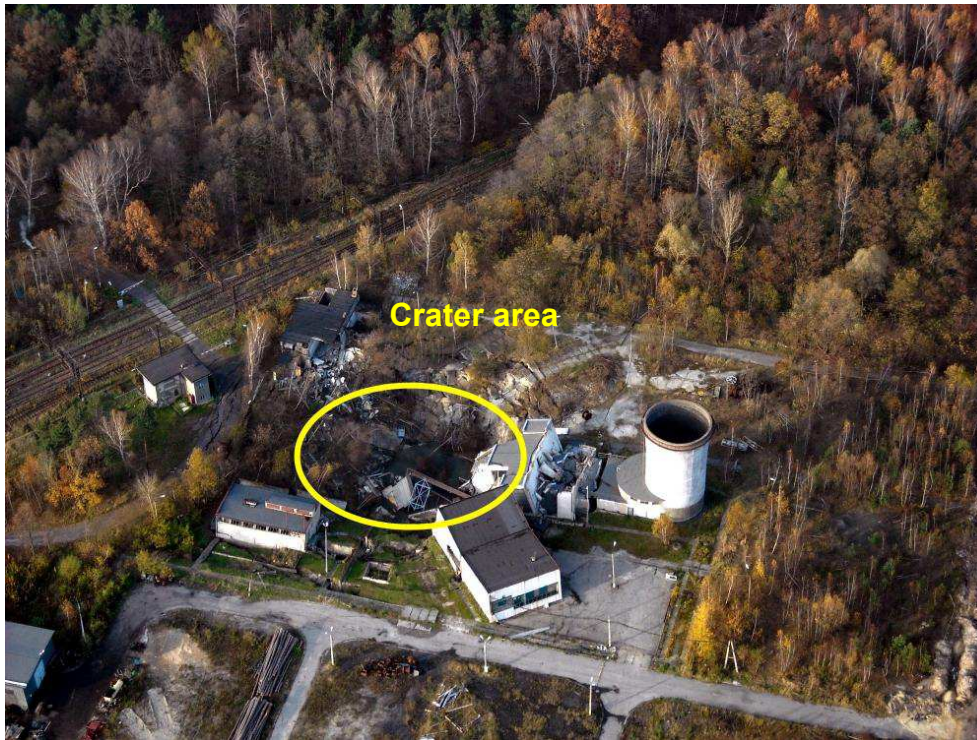
Figure 13 : General view of the scene of the catastrophe of shaft V from the south (Source: GIG / KWSA)
