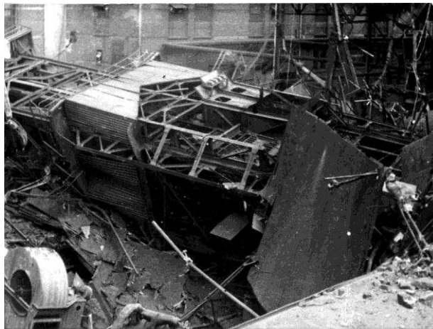
Figure 7 : View of the collapsed headframe (Source: GIG / KWSA)
