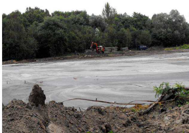
Figure 16 : Final crater fill with building debris mixed with binding material – 31 August 2010 (Source: GIG / KWSA)
