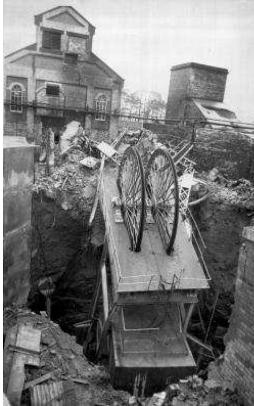
Figure 3 : N°2 Shaft following Collapse (Source: MRSL)
