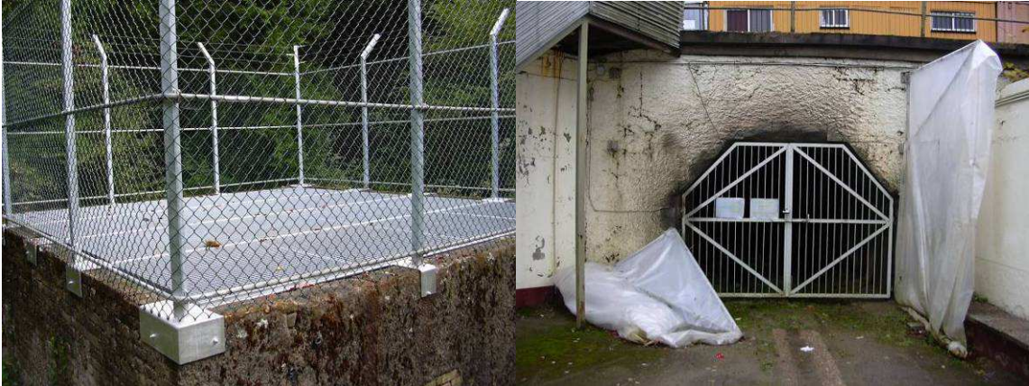
Figure 3: François shaft (left) and Algrange adit (right).
