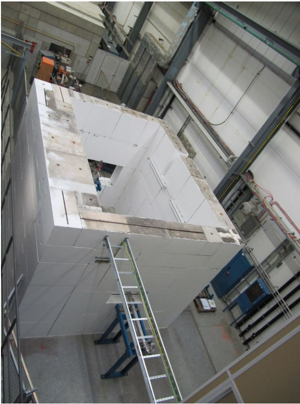
Figure 6: Radiation protection shelter in front of the HLI shelter in December 2012.
