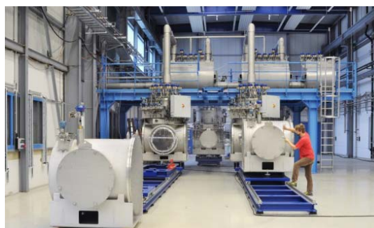
Figure 2: Ground floor: The two right-hand test benches. First floor: The two distribution boxes and the multi-purpose terminal.
