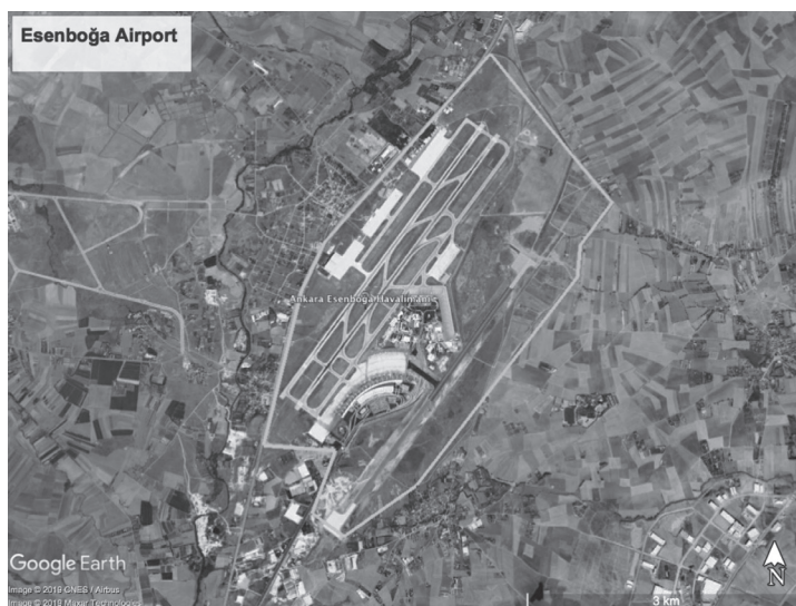
Figure 1. General view of Esenboğa Airport
