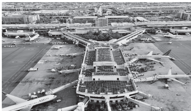
Figure 3. Solar panel installation at HNL airport on Terminal 2 (HDoT, 2019)
