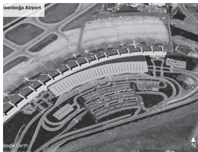
Figure 5. Esenboğa Airport Terminal Rooftop Area
