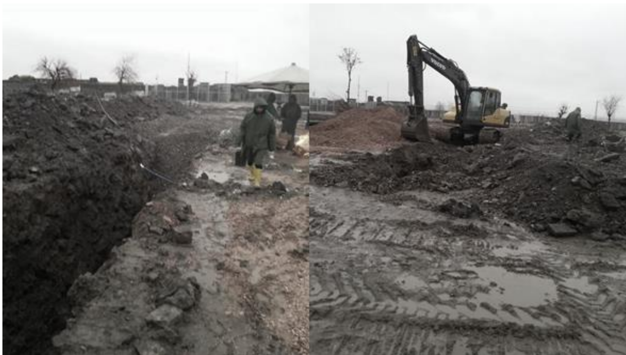
Figure 5. Images from the drinking water line laying Suriçi after urban transformation (2018) [14]
