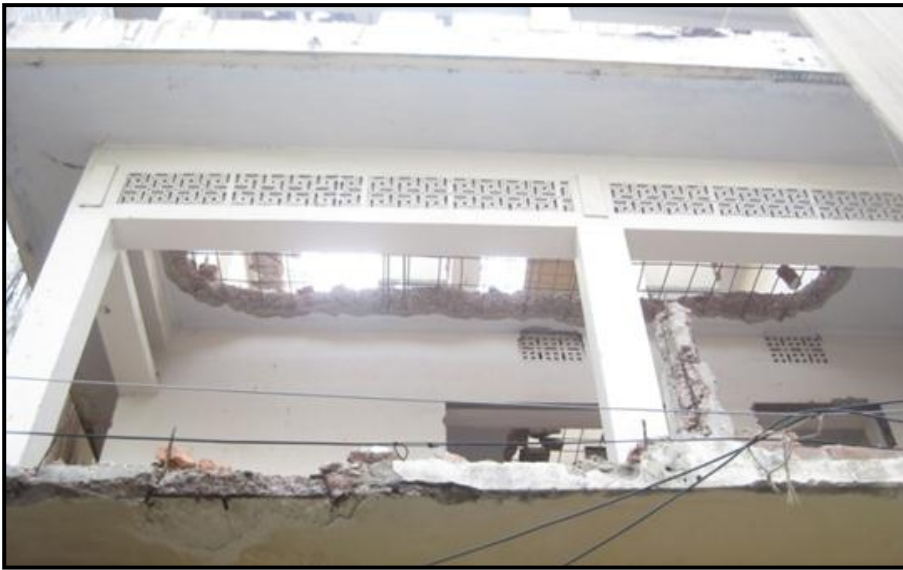
Fig. 3.2 Building under Demolition
