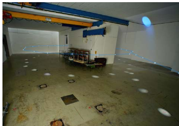
Figure 1: The completed cave for the installation of CRYRING@ESR. The light spots on the floor indicate the position of the bending dipoles and straight sections. The future beam path is marked with the blue line.
