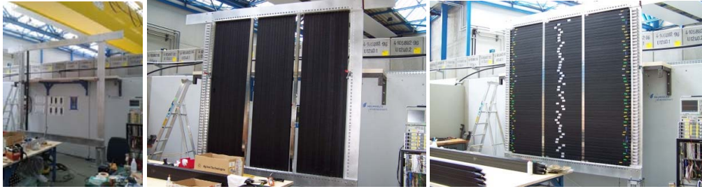
Figure 2: The Photographs show (left to right) an empty double-plane frame, a frame after mounting of the vertically oriented bars and after installation of the support structure for the horizontally oriented bars and a frame after assembly of all scintillator bars prior to mounting of PMTs.
