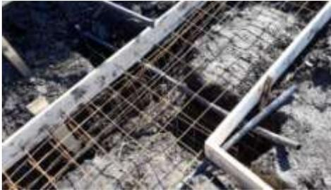
Fig. 8 Welded mesh detail (*original*)
