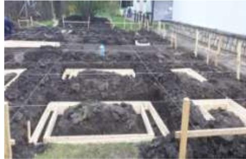
Fig. 7. Belt formwork (*original*)
