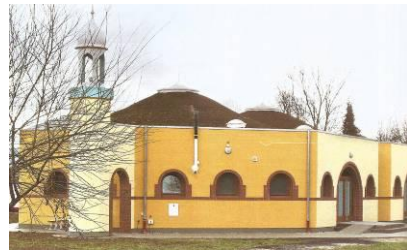
Fig. 10 Mosque with two domes, built entirely of unfired clay blocks covered with earth and grass SII, arch. Gernot Minke, Wabern, Germany, 2007 (World Heritage, 2012)
