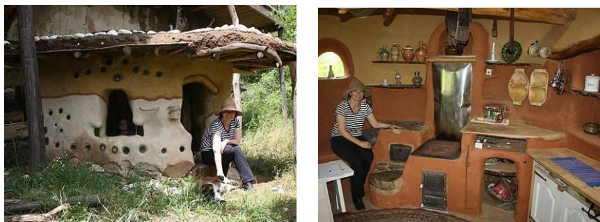
Fig.7 Bio House, Sasca, Caras Severin, Romania ( http://agointel.ro )
