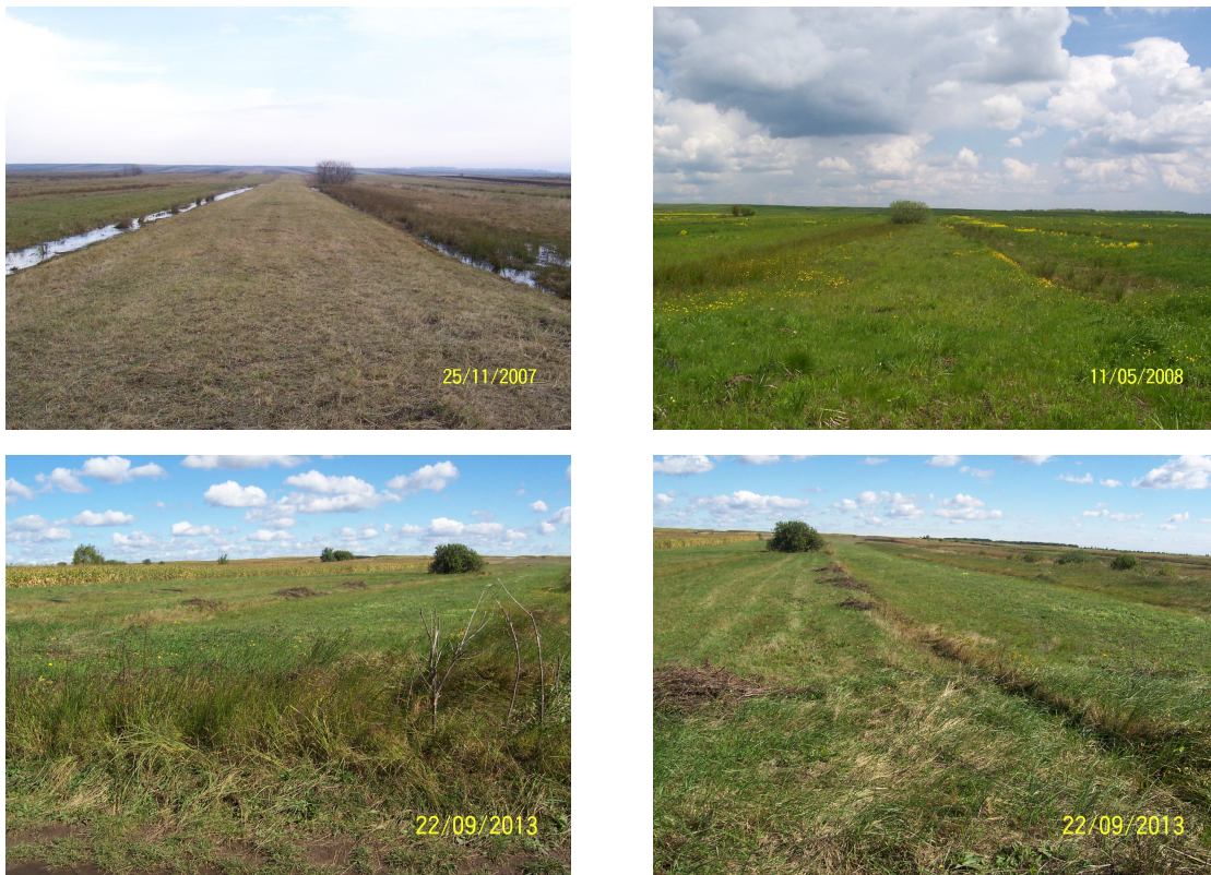
Figure 4 Water stagnation and the installation of hydrophilic plants
