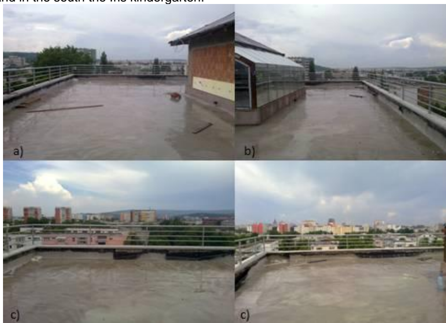
Fig. 2 The roof before rehabilitation
