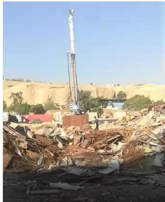
Figure 109- The Damage of the Market After Removing Parts of it by Force (Author's Footage, 2020).
