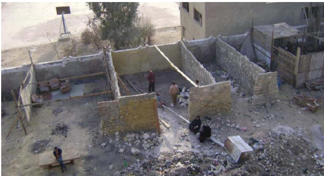
Figure 41- Rebuilding Souq Al-Tunsi With Bricks (Mohamed, 2011)
