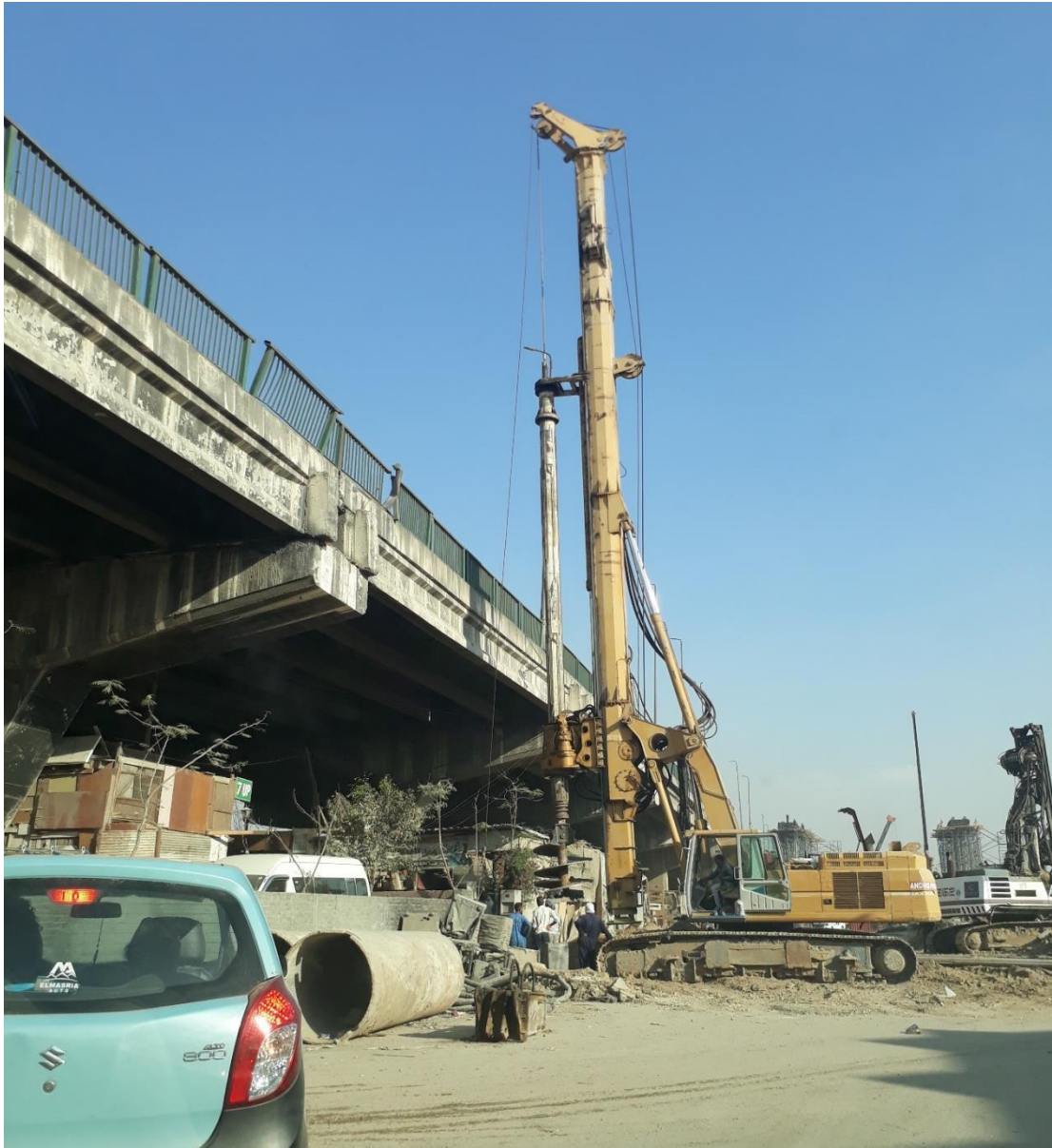
Figure 112- Using a Drill for Building the Bridge Expansion (Author's footage, 2020).
