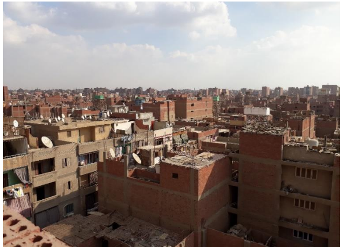
Figure 35- Aerial View on Saft Al-Laban Informal Community (Author's Footage, 2020)
