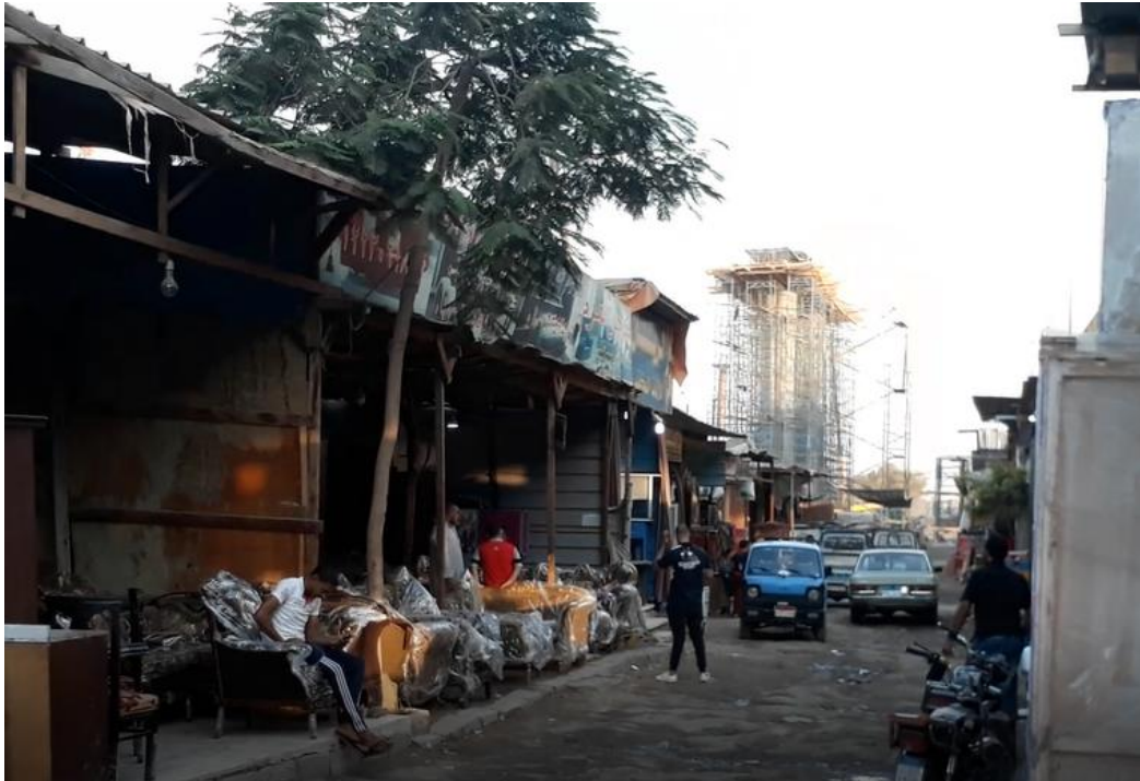
Figure 111- The Expansion of Al-Tunsi Bridge (Author's Footage, 2020).
