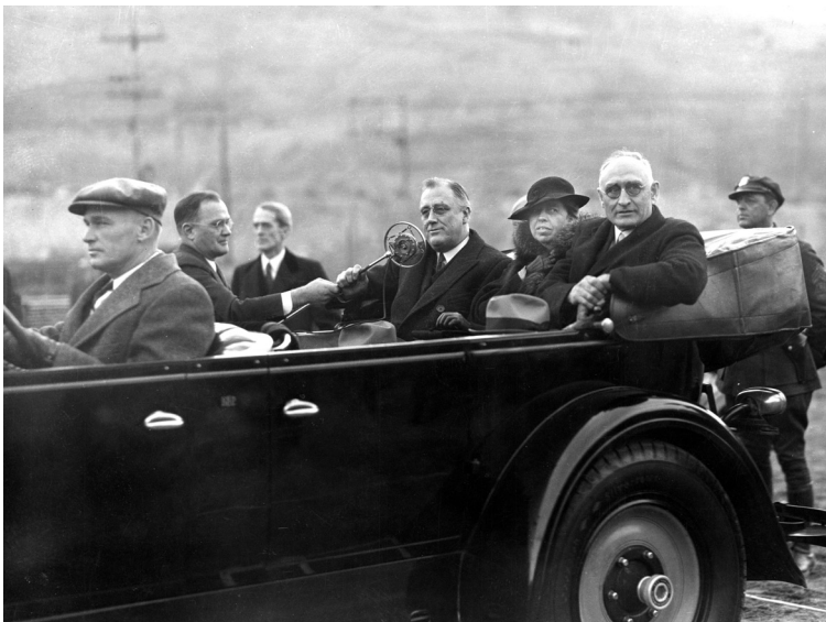
Figure 3.1. Franklin D. Roosevelt, Eleanor Roosevelt, and Arthur E. Morgan (first chairman of the Tennessee Valley Authority) visit Norris Dam construction. (Photo courtesy of the Tennessee Valley Authority.)
