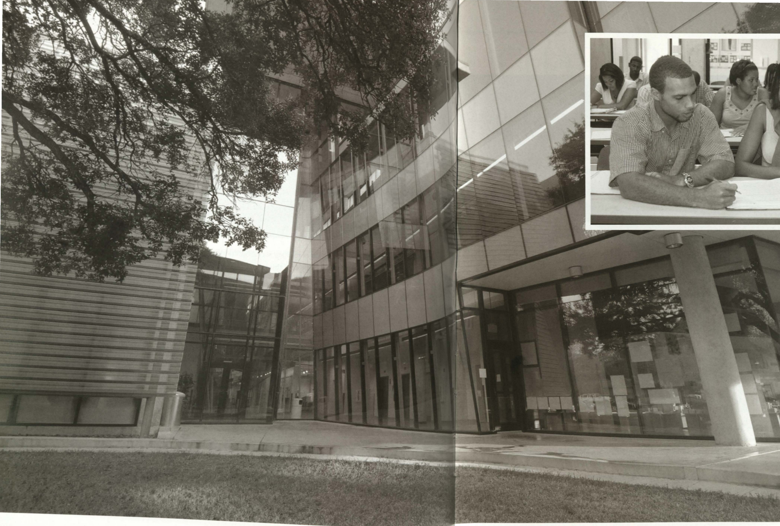
Academic buildings such as the Nathelyne Archie Kennedy building, home of the School of Architecture, house state-of-the-art classrooms and laboratories needed for students to complete their academic goals.
