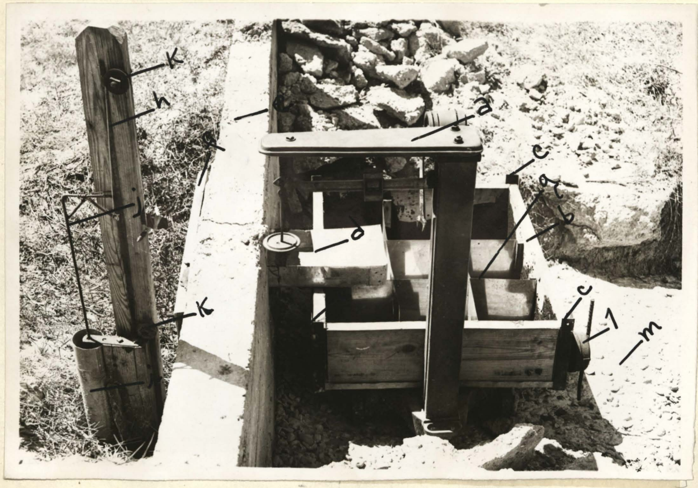
Fig. 4. Weir and Measuring Device
