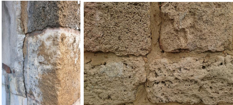
Fig.1: Pictures of the damaged historical sandstones in Tyre old city, where on the left the efflorescence case is presented, while on the right the cavities are formed due to the sub-efflorescence phenomenon, taken in January 2022.
