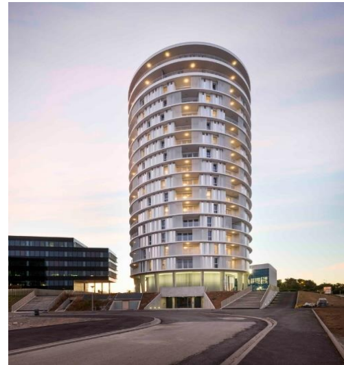
Fig.20: exterior photograph of “Tour Lumiere”
