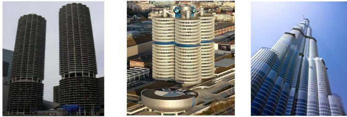
Fig.6: Examples for circular geometry in buildings Source: "Cylindrical Surfaces for Social Significant Architectural Projects, 20 th ".
