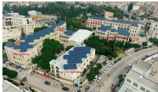
Figure (2): PV installed systems on roof tops of some of PTUK buildings.
