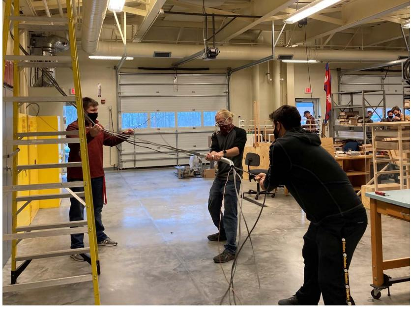
Figure 4: Pulling wire through conduit
