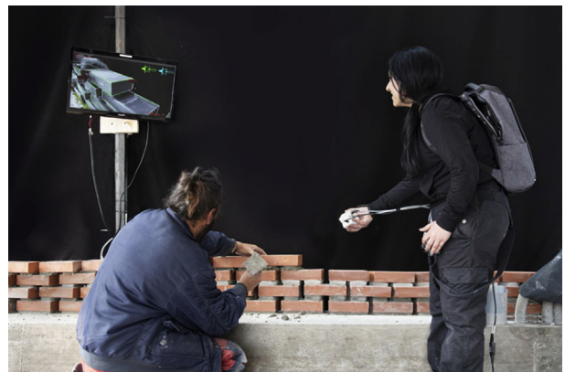
Fig. 10 Bricklayer and assistant’s hands at work on the Kitrvs winery brick skin, © Gramazio & Kohler ( https://gramaziokohler.arch.ethz.ch/web/e/projekte/371.html ).
