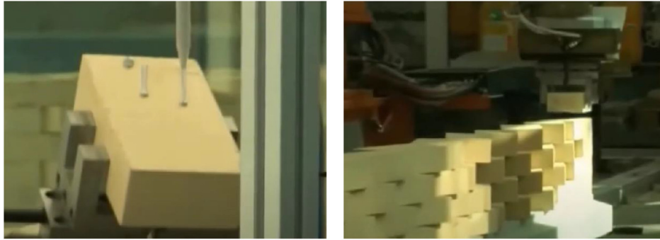
Fig. 12 Bricklaying as reinterpreted by automation, the construction of the Gatenbein winery brick modular panels, © MuDA ( https://www.youtube.com/watch?v=FhL-hWPpnzA ).
