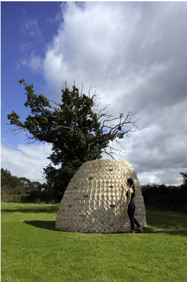
Fig. 15 The subtle angle change of the brick arrangement is highlighted with direct sunlight.
