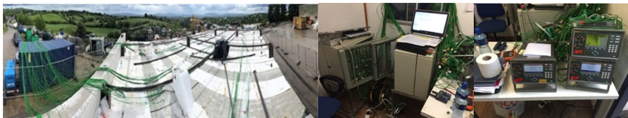
210 211 Figure 5: Extension cables for data sensors and data loggers
