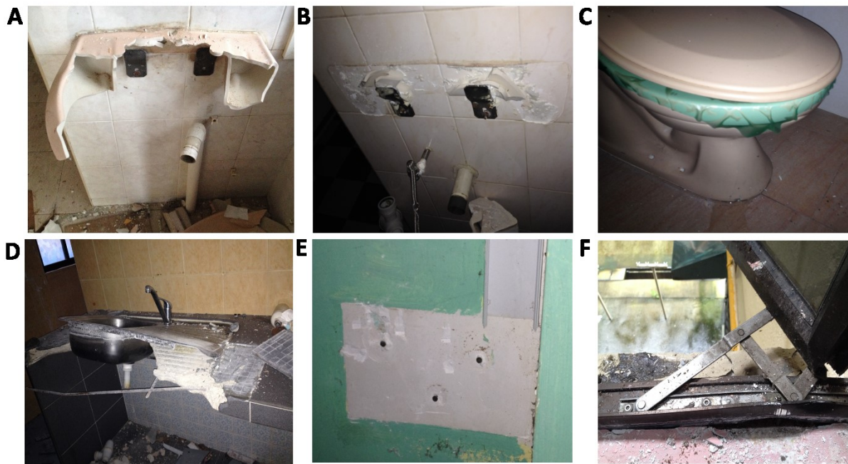
474 Figure 6. Examples of avoidable behavioural practices which lead to breakage of building 475 components during mining namely A. wash basin with white Portland cement (seen in B), C. 476 (unnecessary) nails and white Portland cement at the base of toilet bowl, D. concrete below 477 kitchen basin, E. nails instead of screws in electric boards F. concrete layer below window 478 frame
