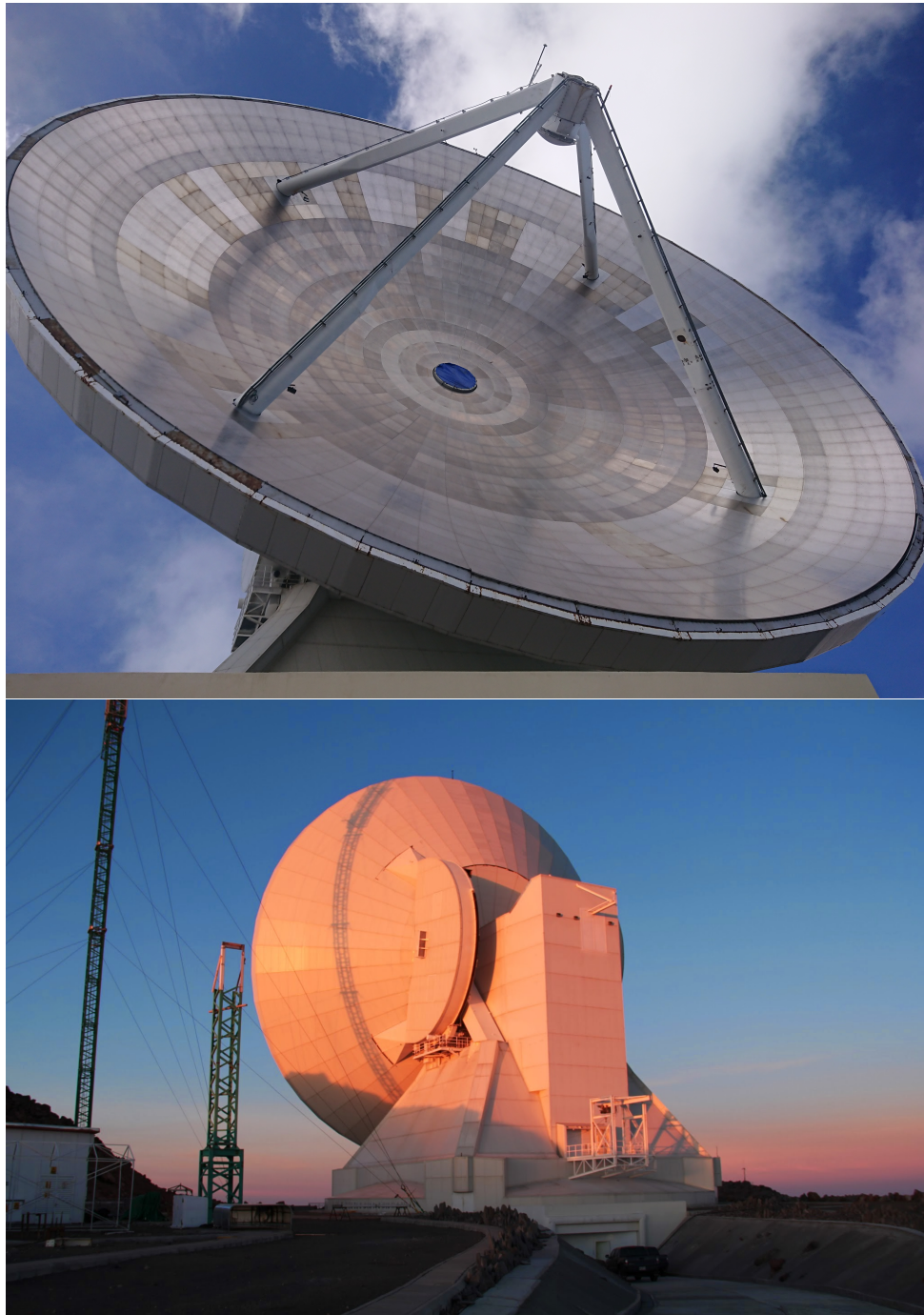
Figure 1. (Above) The 50-meter diameter Large Millimeter Telescope showing the primary reflector containing 180 high-precision surface segments distributed in 5 concentric rings (with 12, 24, 48, 48 and 48 segments respectively). The inner 32-m diameter (rings 1 to 3) of the primary reflector is located interior to the tetrapod legs (in ring 4) that support the 2.7m secondary mirror and hexapod. (Below) The rear-view of the telescope reflector, the ballast cantilevers and the 25-m high building (tower) that contains the elevator to access the drive control units for the major electro-mechanical systems, the telescope control room, and the receiver back-end rooms and main receiver cabin for the scientific instruments. All of telescope structure is enclosed in thermal cladding. The concrete ramp that leads down into the telescope basement, providing access to the telescope, can be seen in the foreground.
