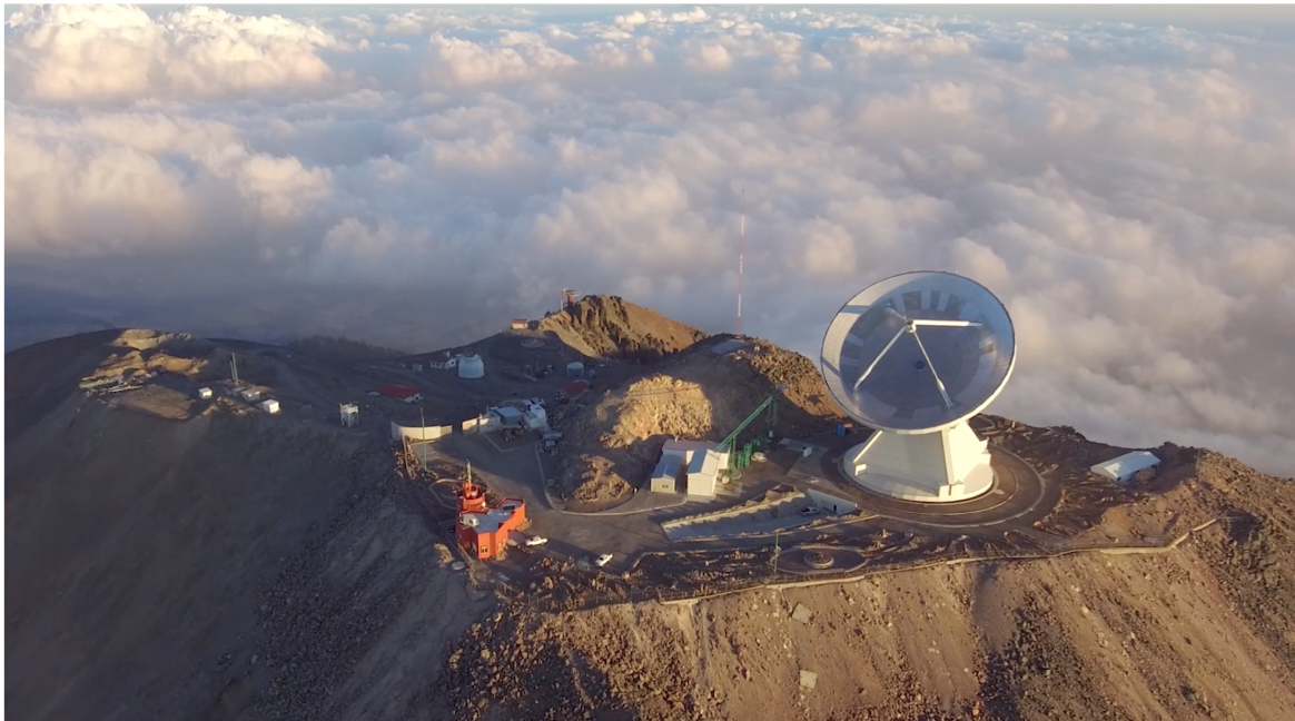
Figure 2. Aerial view (late afternoon) of the summit of Volcán Sierra Negra (altitude 4600m). The site shows the LMT pointing north. The electrical substation, workshop and metrology building can be seen to the left of the telescope, and above the ramp. The green tower-crane (in its lowered position) provides access for installation and maintenance to the secondary mirror, hexapod and segments of the primary reflector (M1), as well as providing the platform to conduct photogrammetry measurements of M1. The red building is occasionally used as a visitor center, and the meteorological equipment including the 225GHz radiometer and external cameras are installed on the roof area of this building. Multiple lightning protection towers are distributed around the summit site.
