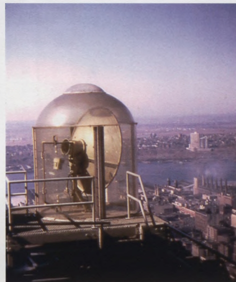
One of 4 Microwave Receiver sites on the RCA Building. NBC had two positions, the northeast and southwest corners. ABC also had two on the opposite corners. If needed we could use each other's positions. In the many years I worked on the "roof" I never met an ABC operator.
