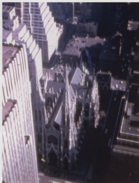
St. Patrick's Cathedral from the northeast microwave dome.
