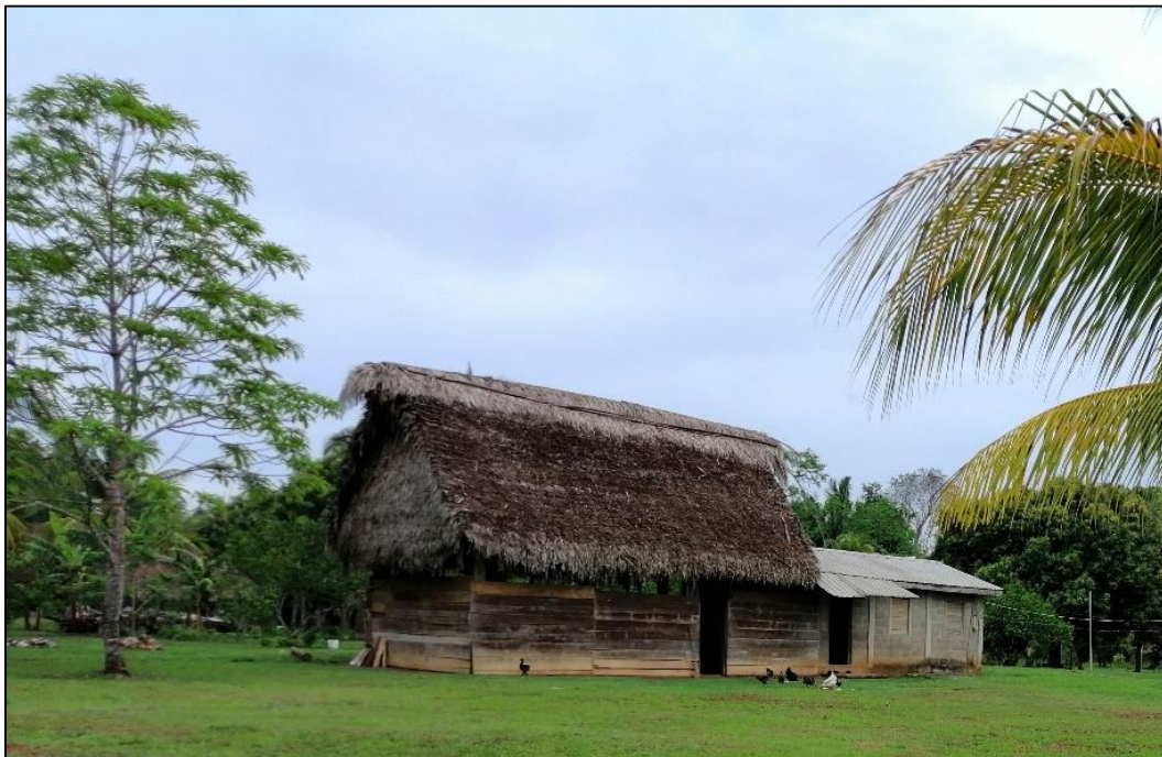
Figure 27: Construction of a typical home at Indian Creek.
