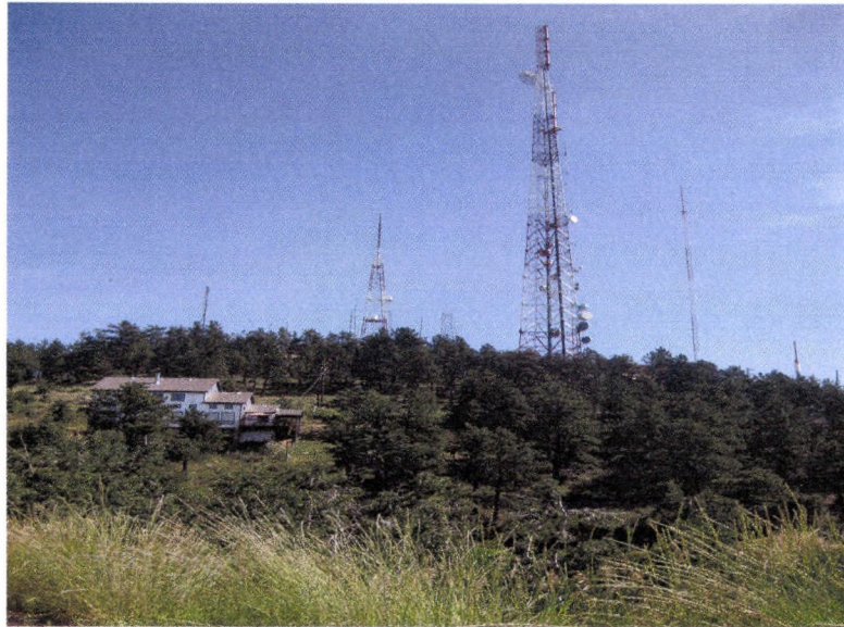
Figure 2 - Radio and TV Broadcasting Towers on Lookout Mountain
