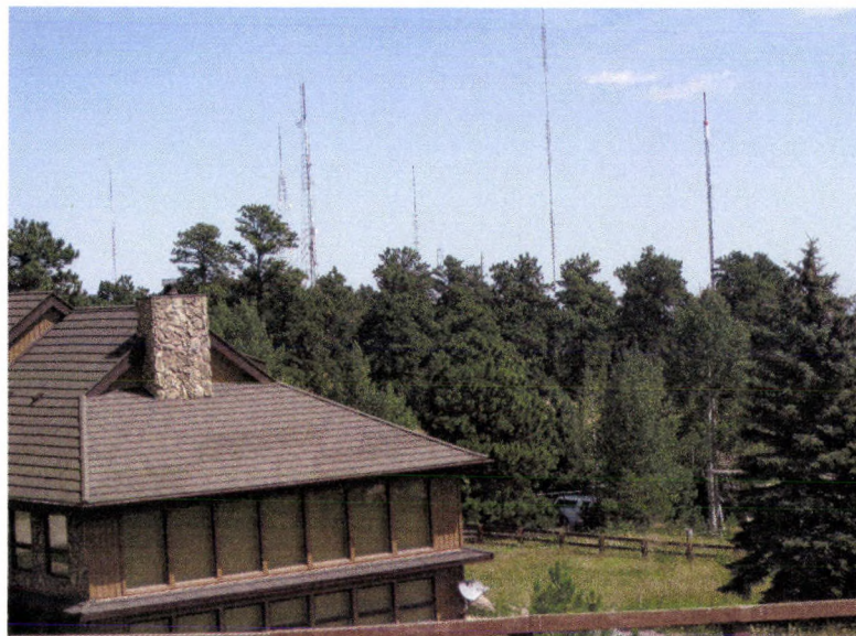
Figure 3 - Radio and TV Broadcasting Towers on Lookout Mountain
