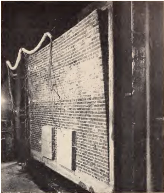
Unexposed face of 305 mm thick clay brick wall after fire endurance test
