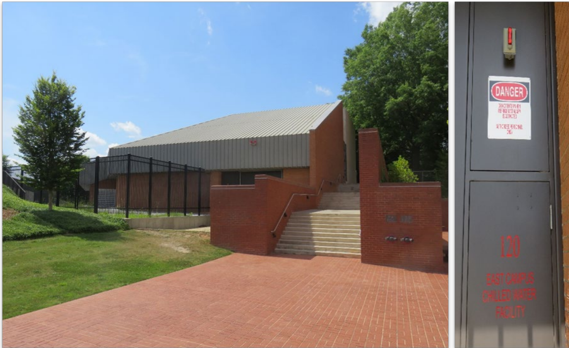
Figure D-8: East side chiller plant photographs.
