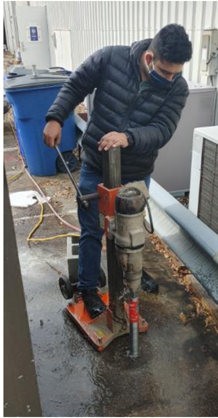
Fig 4.4: Drilling out a concrete core from the pavement
