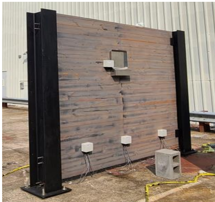
Fig 4.13: Sensors installed on noise barrier for long term monitoring (Rear View)
