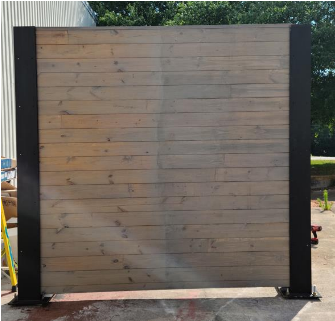
Fig 4.10: Installed noise barrier at BEL Lab, Pendleton SC
