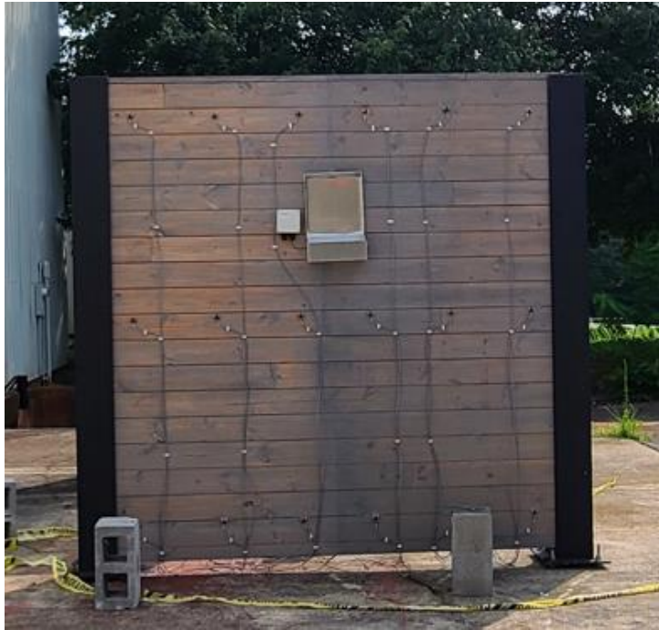
Fig 4.12: Sensors installed on noise barrier for long term monitoring (Front View)
