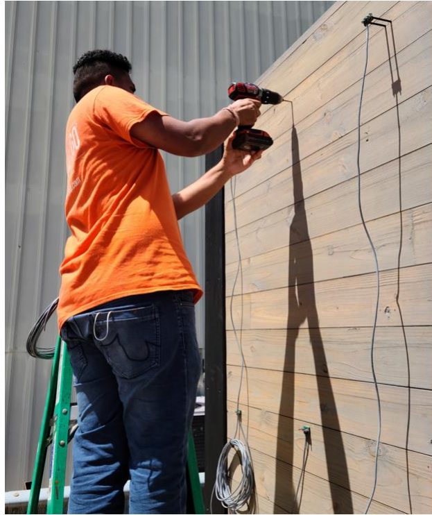
Fig 4.11: Installing PMM's at the required depths in the CLT panel
