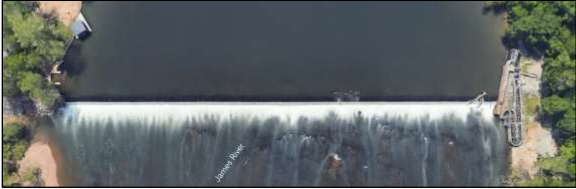
Figure 34. Overhead view of the existing Boshers Dam site.
