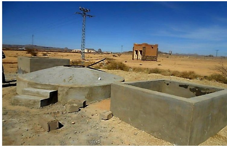
Figure 10. Biogas digester with a capacity of 15m 3 installed at Tamanrasset city (Southern of Algeria) (K. Benaissa et al., 2017(a),(b))
