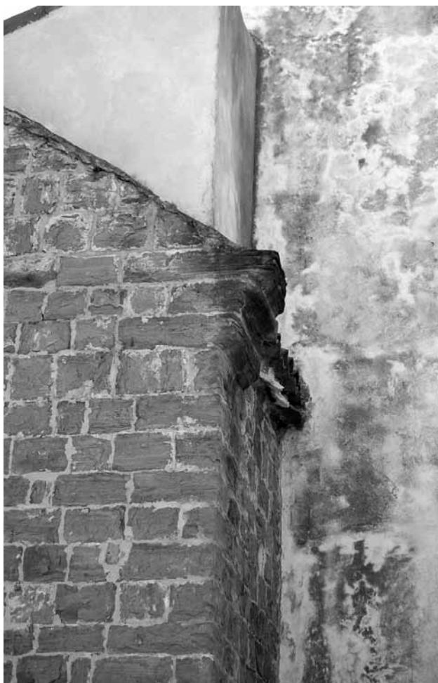
Sl. 32: Piran, minoritska cerkev, venčni zidec na severnem vogalu prezbiterja (foto: M. Oter Gorenčič). Fig. 32: Piran, Minorite church, cornice in the north corner of the presbytery (photo: M. Oter Gorenčič).
