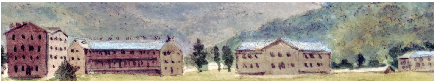
The South Barracks is the second building from the left in this 1830s painting by John Ruibens Smith. The 1817 North Barracks is on the far left, and to the right of the South Barracks are the 1815 Academy and the 1815 Refectory (Mess Hall). Source: Library of Congress
