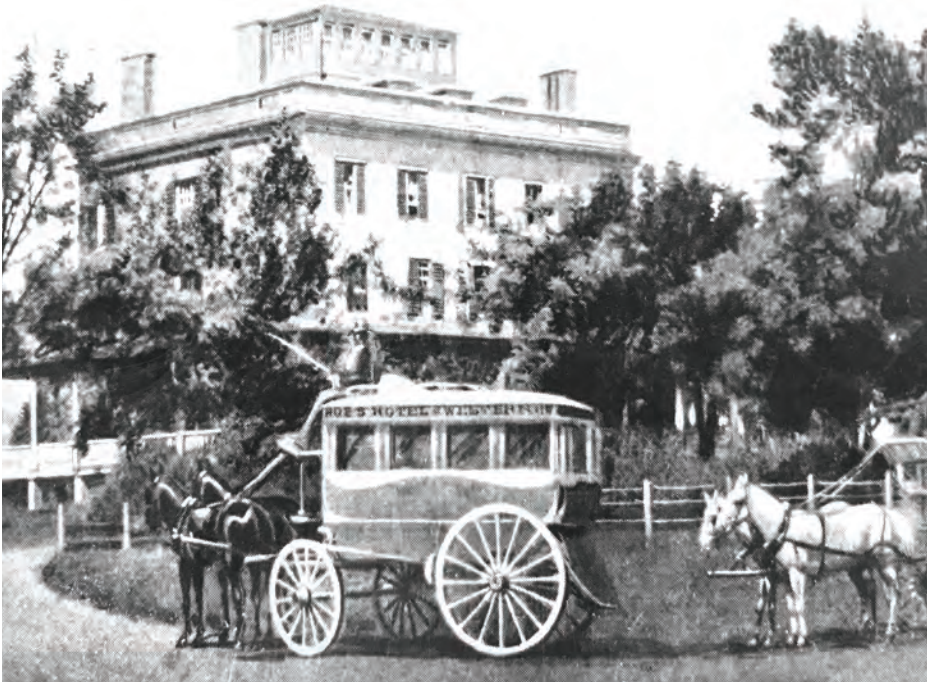
Before the 1850s, guests would climb or ride up the hill from the dock. From 1850 onward, guests arriving by steamer would stop at Cozzens' Landing in Highland Falls or later in the century at what is now known as South Dock. Omnibus carriages, as shown in this image from the Civil War era, would then take them to the Hotel. Note that it says Roe's Hotel West Point and not the West Point Hotel. After 1850, rail passengers on the east side of the river were ferried by boats that met the trains. Rail service to West Point did not begin until 1883. Source: USMA Archives
