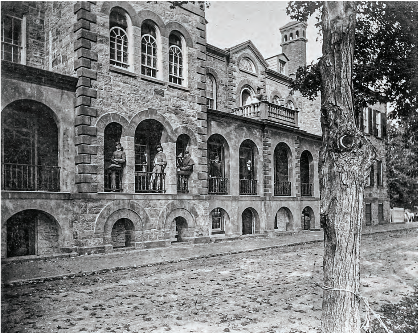
The Cadets' Hospital as it appears in an 1873 class album. The stonework, including the quoins along the edges, bears a strong similarity to Professors Row, the only surviving stone buildings from this era. The rounded Roman arches would have resembled those on the 1815 Academy building also standing at the time of the Hospital's construction and would again be included on the (Old) Cadet Chapel in 1836. Source: USMA Archives
